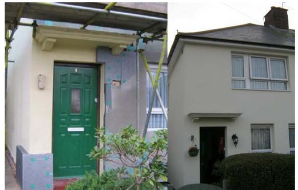
Left: Image of a house during the installation of external wall insulation.
